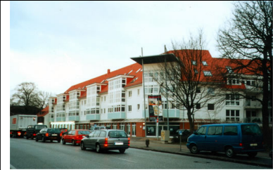
PE / Bau Eidelstedt 100 WE + GW 98
